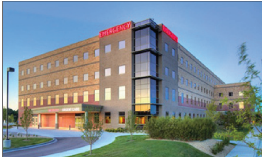
The $17 million, four-story, 158,000 square foot Two Twelve Medical Center in the southwest Minneapolis suburb of Chaska, the largest medical office building to open last year in the Twin Cities metro area, is already fully leased. Photo courtesy of Mount Development Co.
