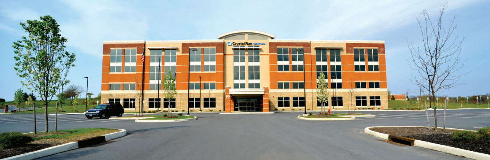
The six-building Crystal Run MOB portfolio includes the 127,000 square foot 95 Crystal Run Road in Middletown, N.Y.
